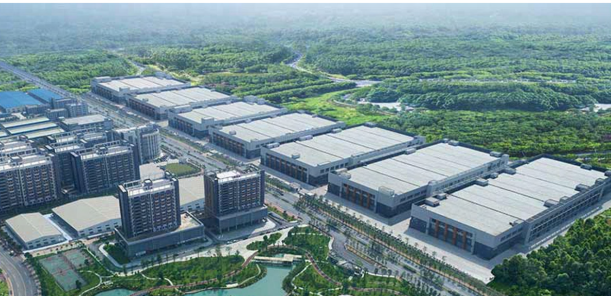
MODERN, LARGE-SCALE MANUFACTURING FACILITIES
